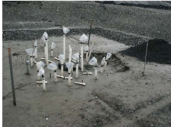
Sinkhole in southernmost cell
