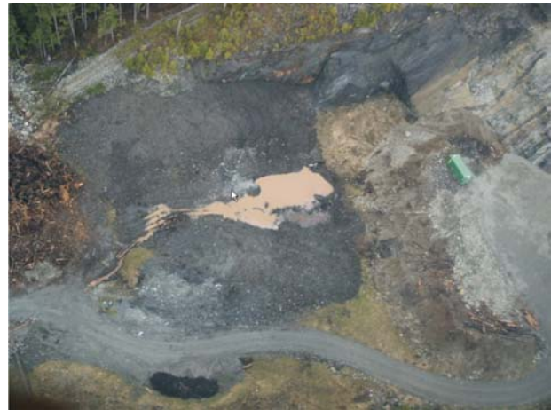
Aerial view of Pit 7.
