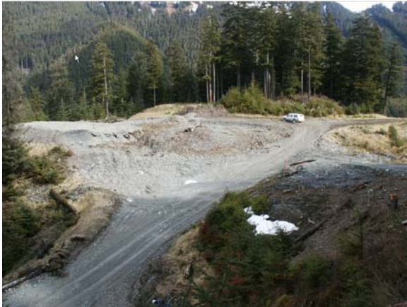
Area at Site 1350 where material removed.
