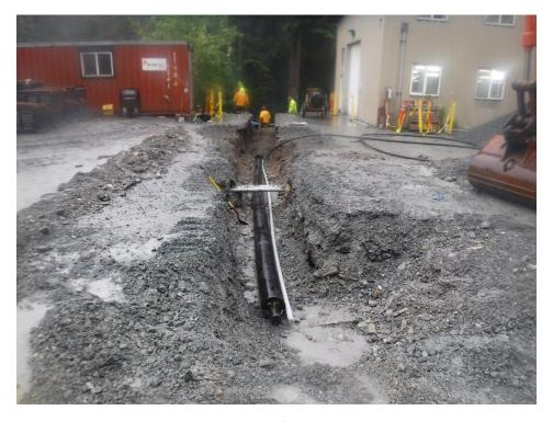
PHOTO 10. New discharge pipe being installed from upper Pond C.
