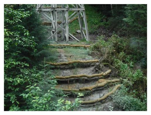
PHOTO 8. New straw wattles on north abutment of Zinc Creek bridge.
