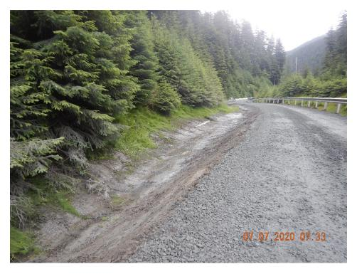
PHOTO 2. Road surface raised to establish a larger conveyance ditch for runoff.
