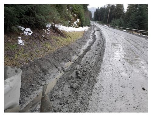
PHOTO 4. Repair of ditch above 3.4-mile bridge following 1 December storm.
