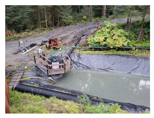
PHOTO 9. New discharge line from upper Pond C. Old piping remains in place as a backup.
