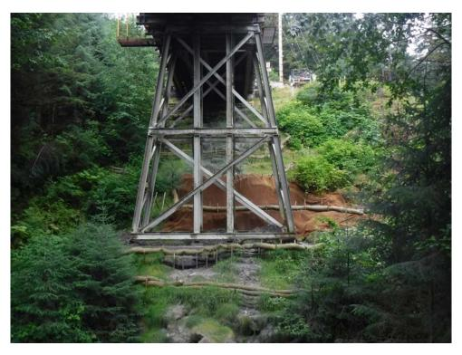
PHOTO 7. New straw wattles on south abutment of Zinc Creek bridge.
