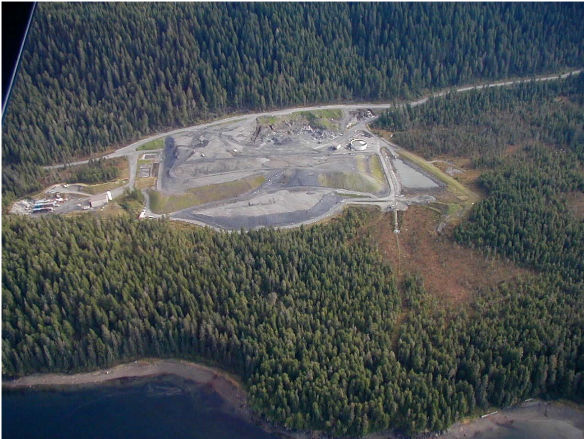
Figure 2.46 Aerial Photograph of Tailings Facility 2001
