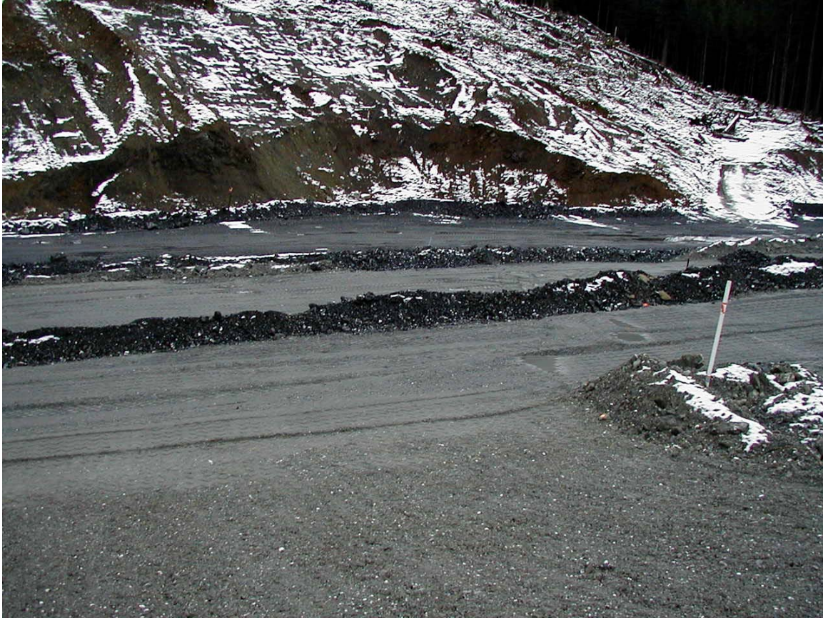
Figure 3.46 Photograph of Site 23 Backslope and Designated Placement Zones
