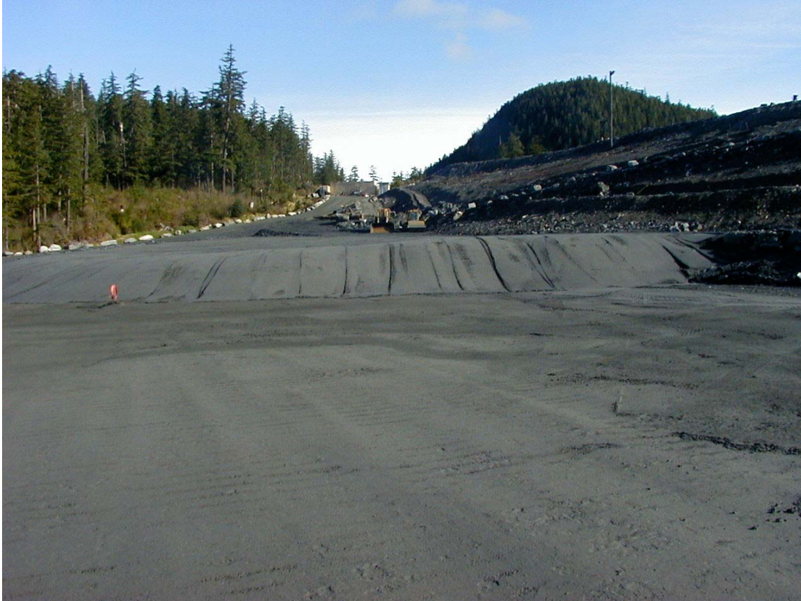
Figure 2.49 Photograph of Compacted West Buttress Tailings
