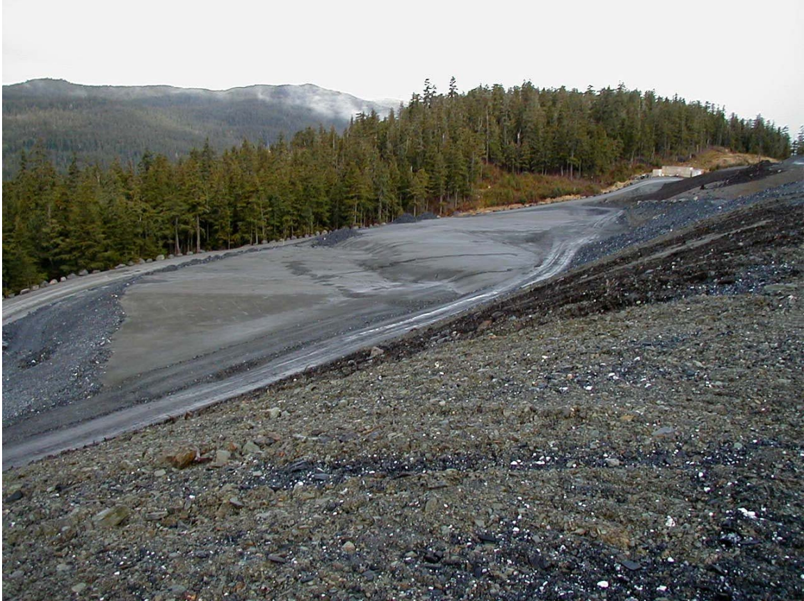
Figure 2.48 Photograph of West Buttress Tailings Placement Area
