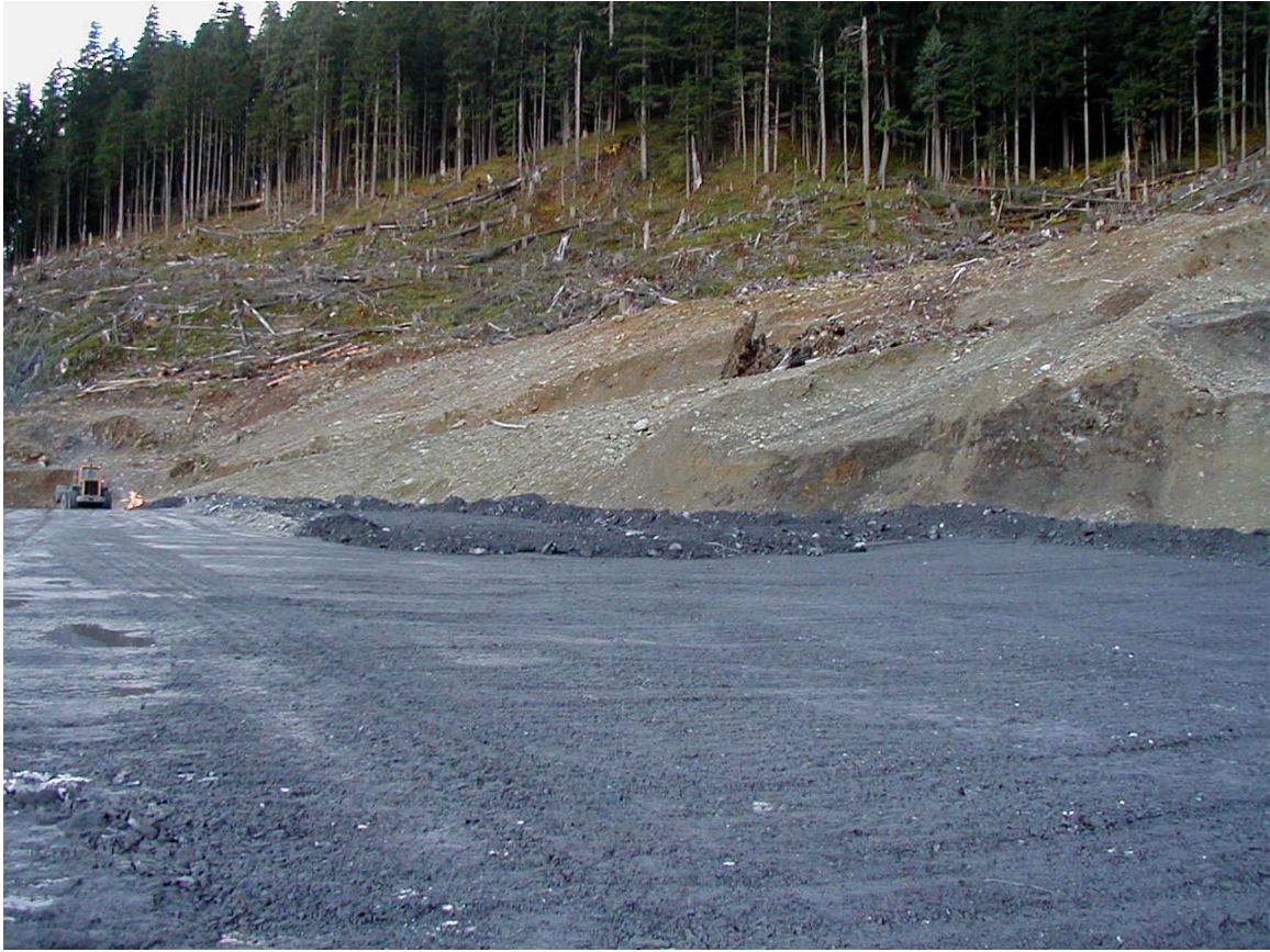
Figure 3.45 Photograph of Site 23 Foundation Preparation
