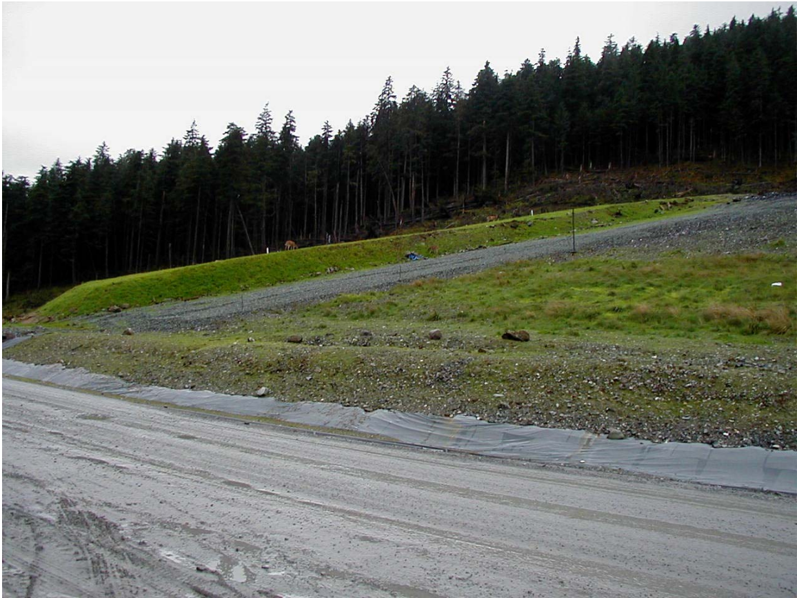
Figure 3.43 Photograph of Site 23 Composite Soil Cover Plot
