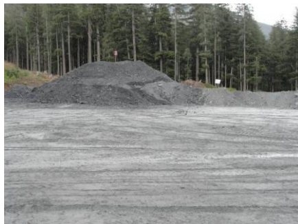
Site 23 - Note: Upper Surface Compacted and Sloped to Drain (no ponding present)
