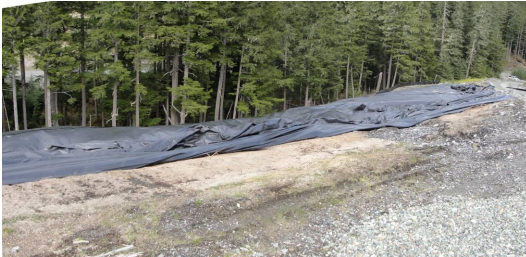
Geosynthetic Cover at Site E
