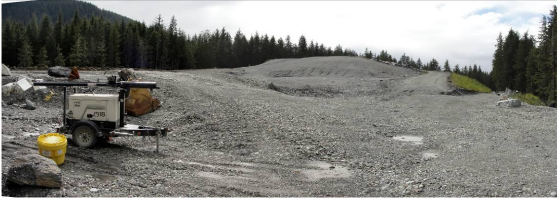
Site E Southwest Aspect at B-Road Entrance
