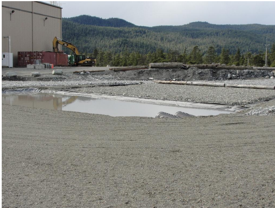
Tailings Disposal Site – Degritting Basin Near Water Treatment Plant
