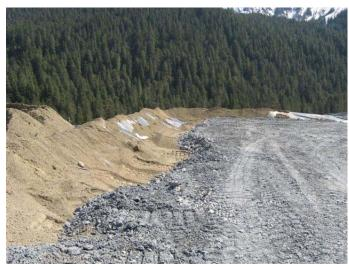
Site 23 pad with sand and class 3 rock over synthetic liner.
