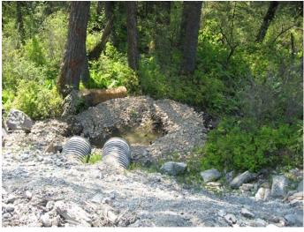
New BMP's to capture sediments from the lined ditch at mile 1.2.
