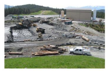
Pond 6 excavation showing the new access road constructed to the right of the photograph to bring rock in from the "clean" road.
