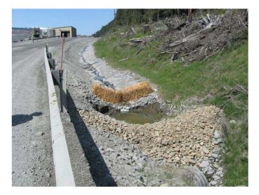
New BMP's to capture sediments from the lined ditch at mile 1.2.
