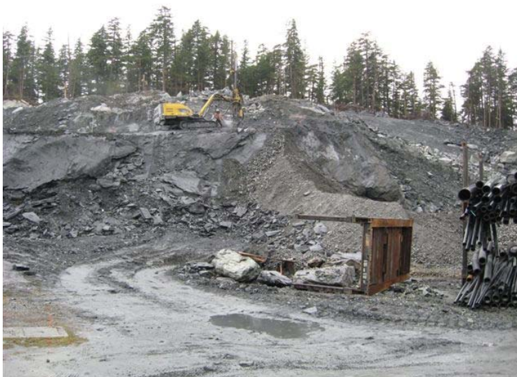
Pit 5 excavation in progress.
