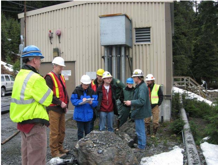
SRK team, agency staff and HGCMC personnel at the water treatment plant / Greens Creek near the mine portal.
