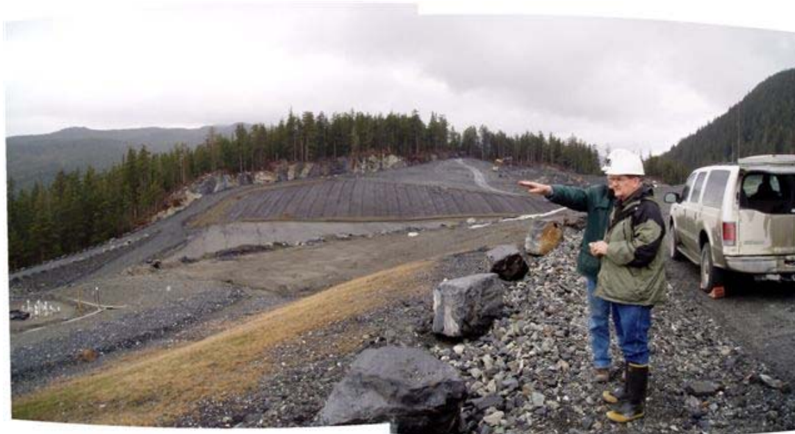
Tailings pile, SRMP cells to the left, Northwest expansion area in the center, Pit 5 to the right.
