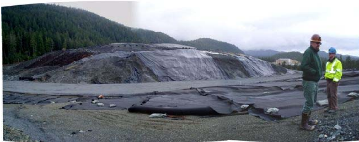
Tailings pile NE corner expansion area
