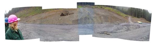
Site 23 – waste placement regime showing progressive placement of a 5-foot layer of Class I production rock at the lower aspect of the facility (upgradient FWMP well #57 in background near treeline)
