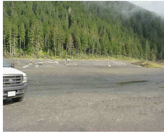
Tailings placement in the lined quarry area
