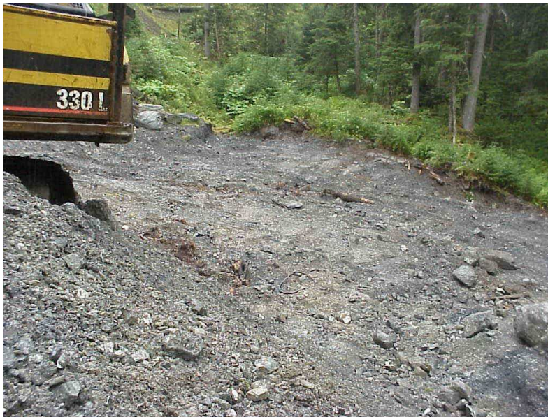
Excavation of Site 960 material
