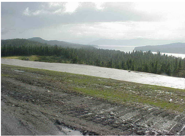
Buttress on the west side of the tailings pile
