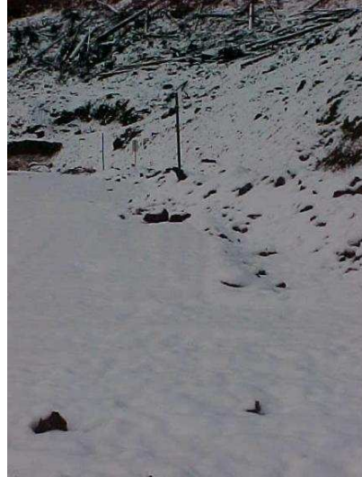
Staked Finger Drains Production Rock Site 23 - Detail
