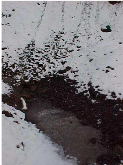
Run-on at Finger Drain
