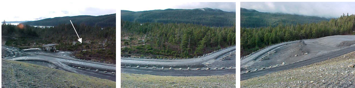
Duck Blind Drain Area Further Seep Drainage Area Northwest Tailings Area (West Buttress) Downgradient Western Area Of The Tailings Disposal Facility
