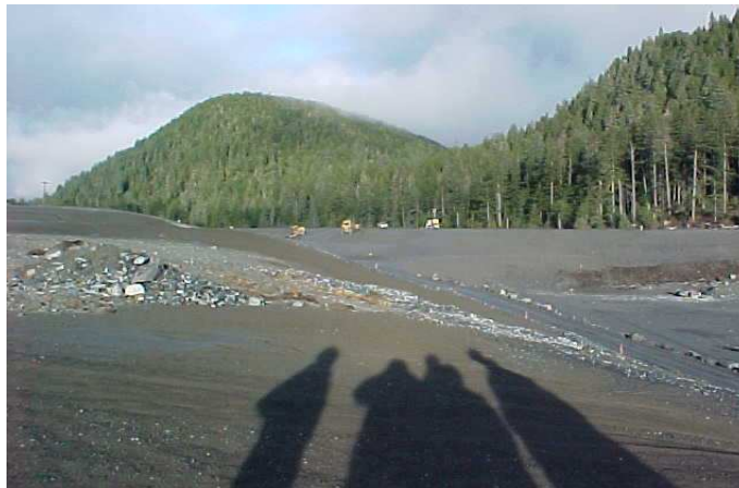
Central Portion (left) and Eastern Portion (right) of Tailings Disposal Facility
