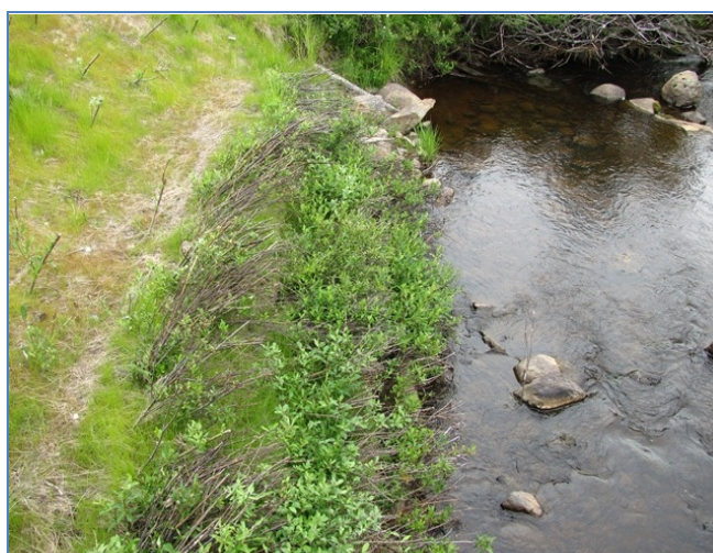
Summer 2012, the same slope as at left, but willows in the brush layers are sending out new growth.
