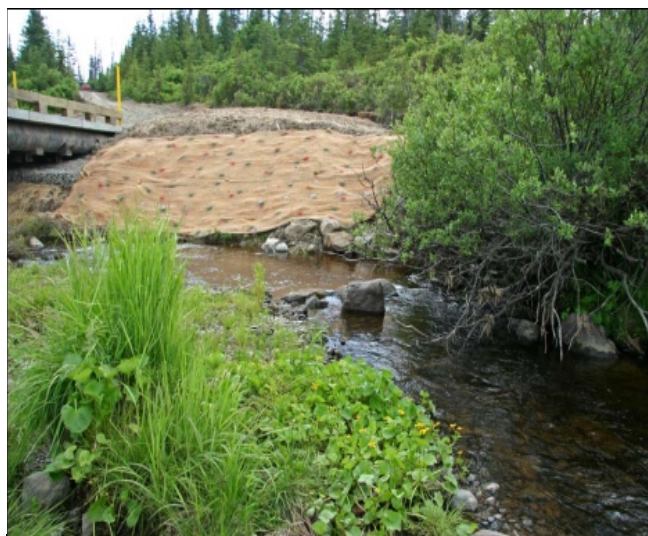
2010, after the bridge was installed. The slope has been covered with geotextile and seeded for the winter.
