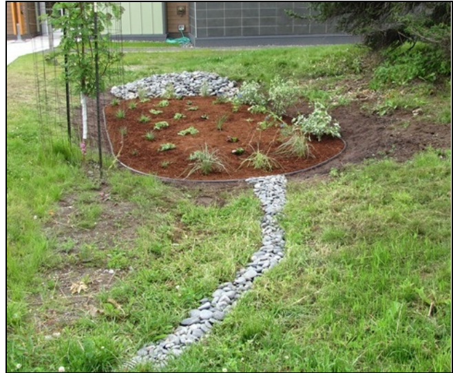
Newly planted rain garden at Homer City Hall. Homer District installed this rain garden to demonstrate a Low Impact Development technique to treat stormwater onsite.
