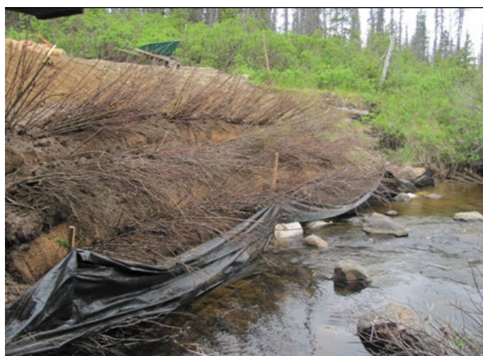
June 2011, the slope was stabilized with a combination of techniques, including brush layering and use of C-125 BN biodegradable fabric with live staking.
