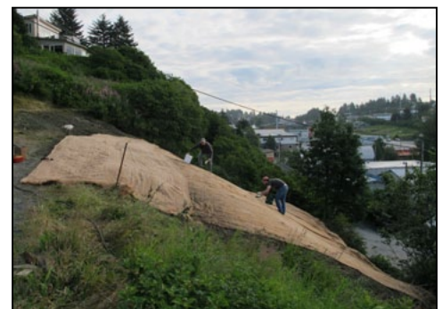
A biodegradable blanket is laid across the site after hydroseeding to prevent further erosion.
