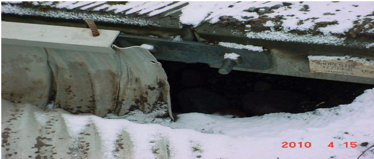
Undermining of the Cold Bay Boat Ramp behind the corrugated half-pipe, near the top of the ramp.
