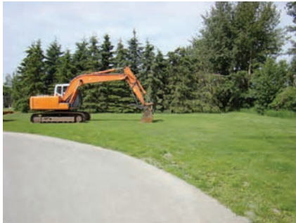
The work begins!
