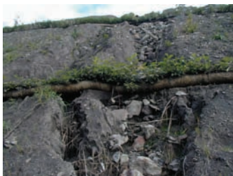
Coir log holds plants in place on steep slopes.
