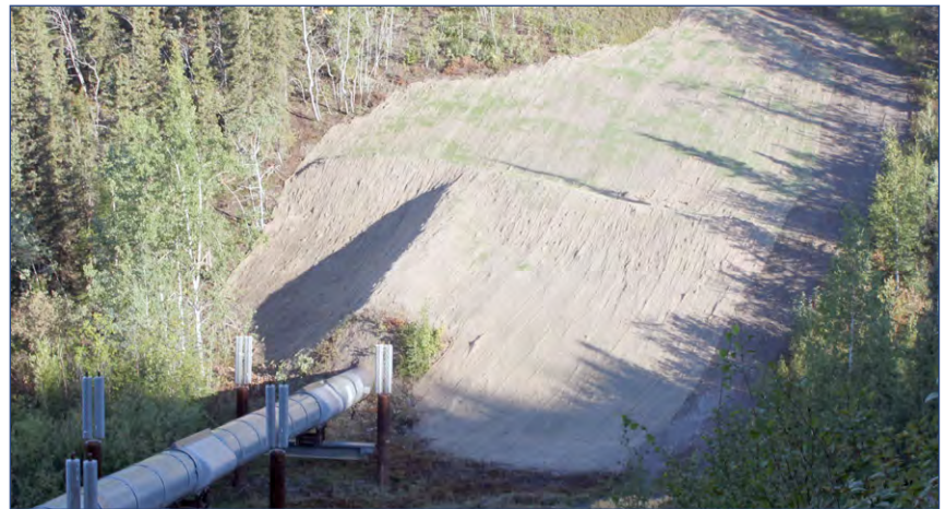
Erosion control fabric is used to establish vegetation cover along the pipeline
