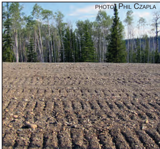
Eagle landfill site capped with topsoil, and ready for fertilizer and seeding. Depressions in the soil create a micro-climate well suited for seed growth.
