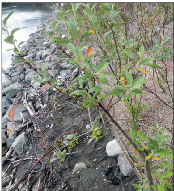
Live willow stakings, erosion control fabric, and armor rock provide slope reinforcement
