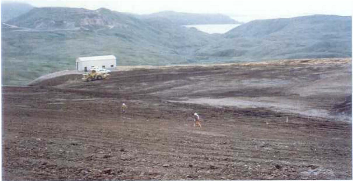
Figure 12. White Alice Landfill after grading, 1997
