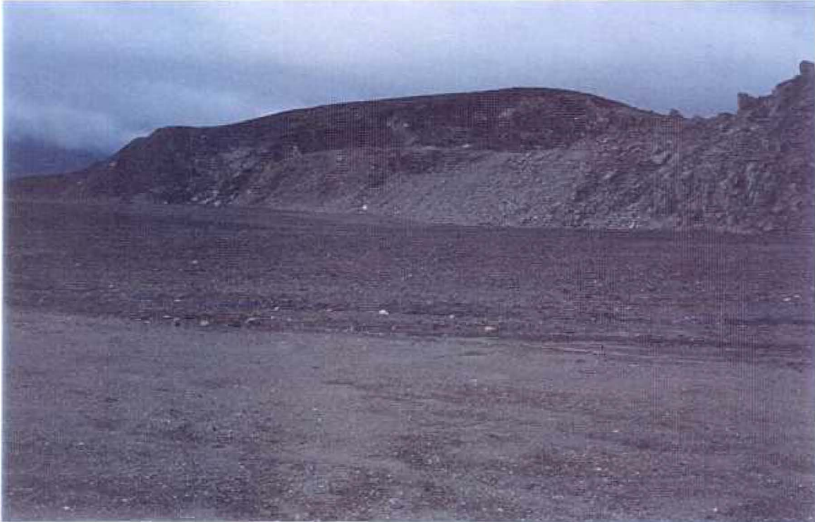
Figure 5. Metals Landfill, 1997, after final grading.
