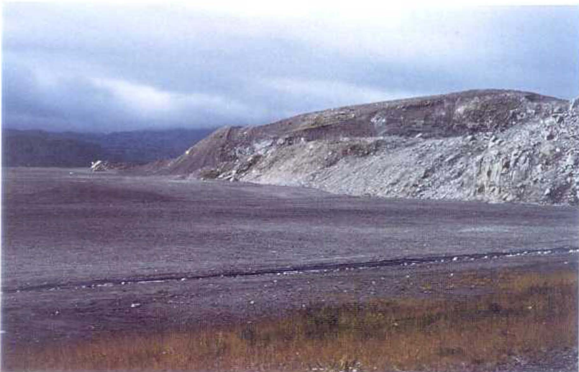
Figure 10. Eroding back slope area at Metals Landfill, 1998.
