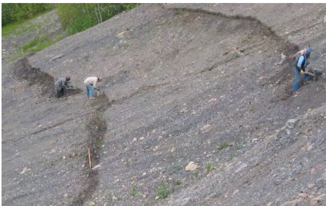
Photo 3. Contour Trenching for Wattle installations
