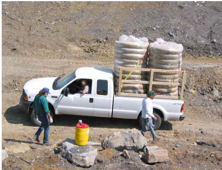
Photo 2. Delivery of Straw Wattle
