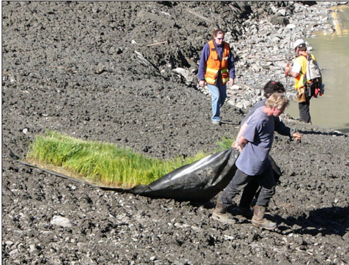
Heavy plastic sheeting facilitates on-site transport of the vegetation mats.
