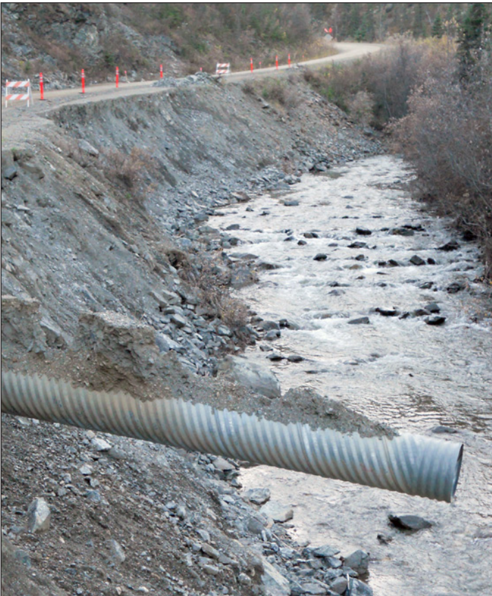
Riverbank erosion exposes a culvert along the Taylor Highway
