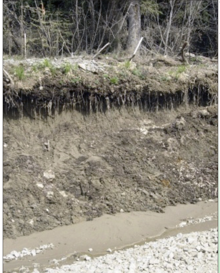
Advanced thawing on a cutslope causing silty runoff to flow into a ditch created using a gravel berm at the edge of the roadway. For further detail on this technique, refer to Alaska DOT Publication No. FHWA-AK-RD-09-11 .
