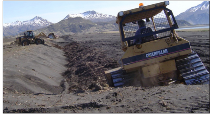
Heavy equipment used to spread topsoil - May, 2006
