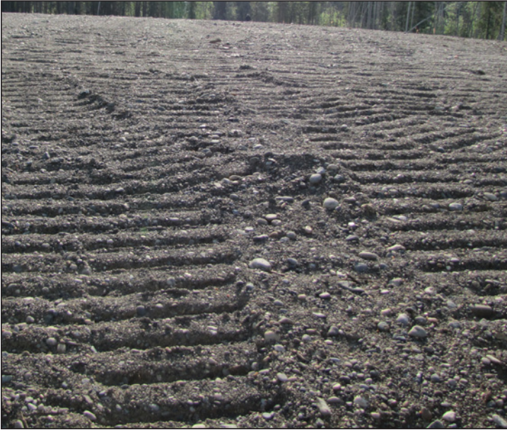
Surface imprinting accomplished using the 'track-walking' technique.
