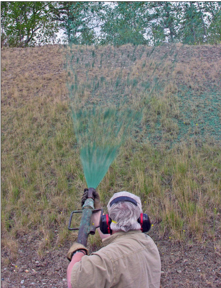
Hydroseeding is used to revegetate slopes that are not easily accessed by traditional seeding equipment
