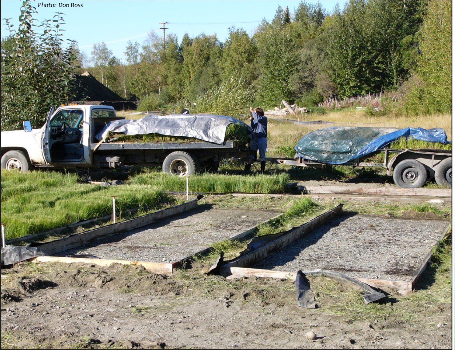
Many techniques exist for revegetation, including pre-prepared vegetation mats
