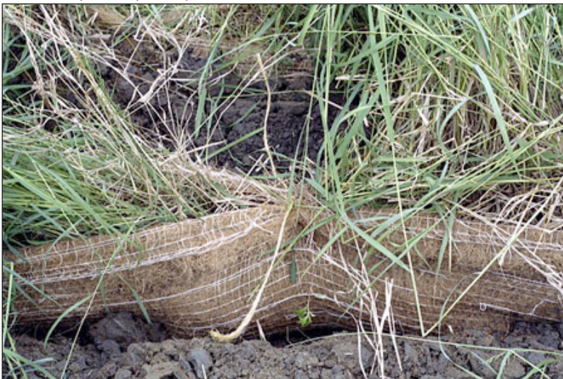
A prepared grass roll, consisting of sod clumps wrapped in a biodegradable fabric, with slits cut in the top for the shoots
