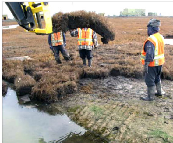
Placement of sod clumps
