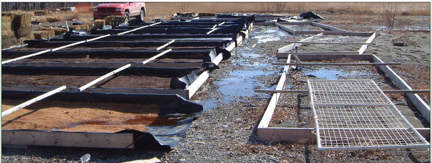
10' x 3' constructed mats framed with dimensional lumber, with thick plastic and erosion control matting used for the base. Only the biodegradable erosion control matting will remain once the mat is deployed.
