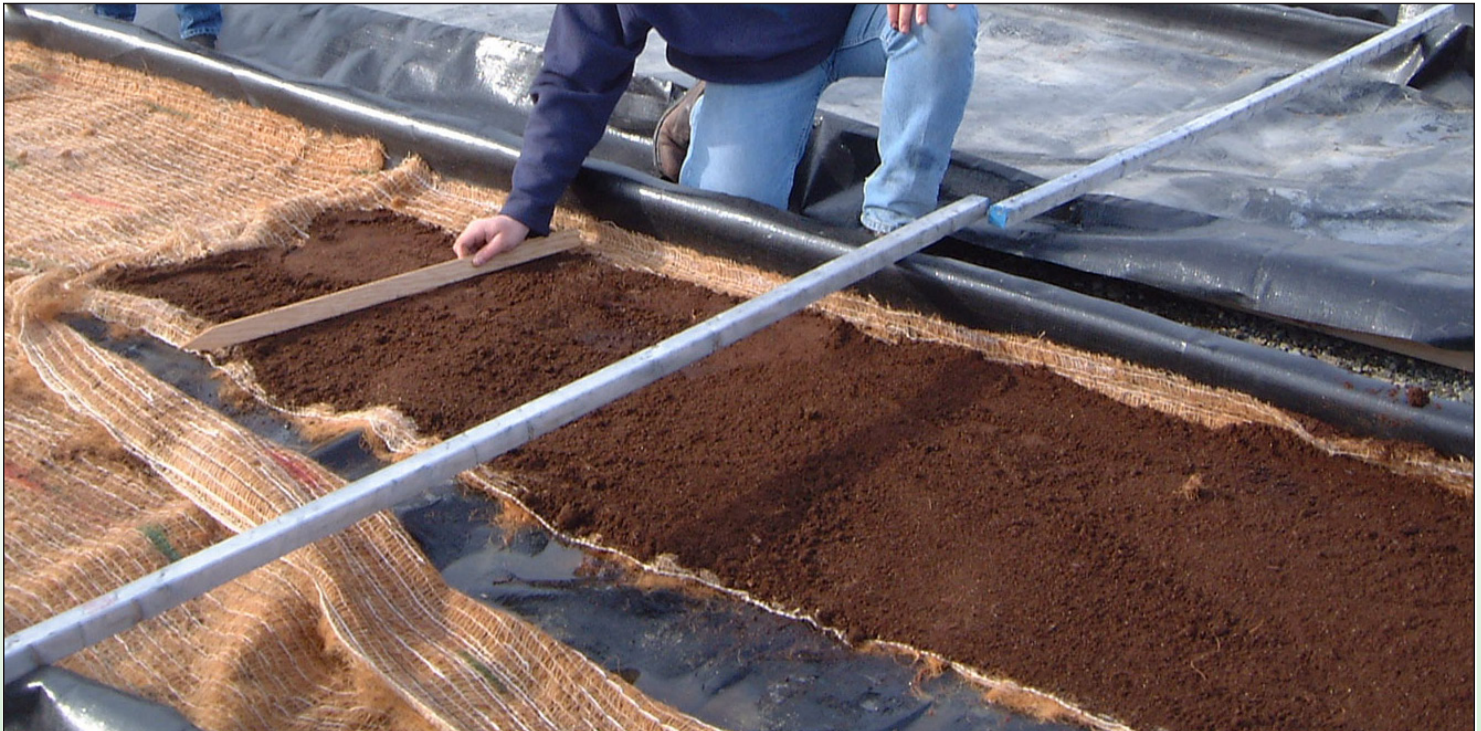
Soil spread on erosion control fabric provides a binding medium for roots.
