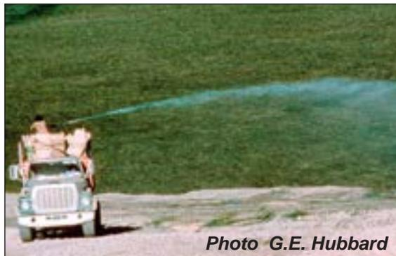
Figure 11: A truck-mounted hydroseeder applies a seed mixture
