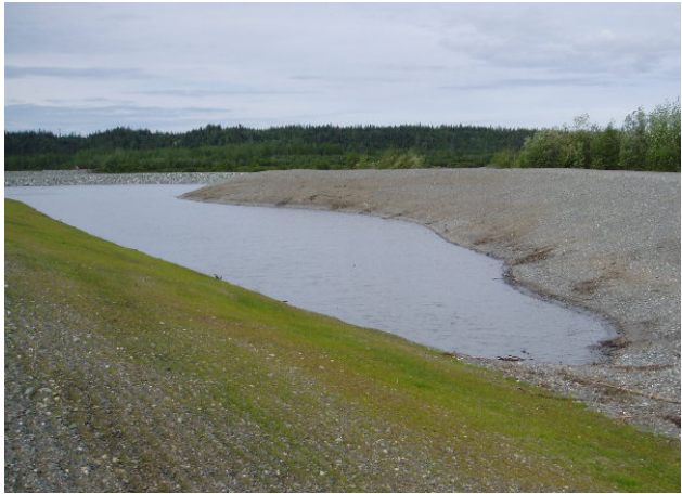
Photo Point 7. June 19, 2006 Northeast Wetland
