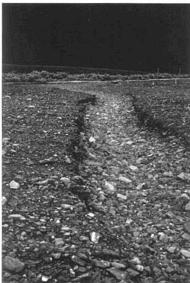
Figure 11. Eroded banks of overflow channel.
