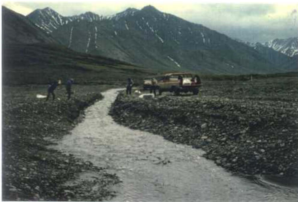
Figure 3. Overflow channel being planted with willow sprigs.
