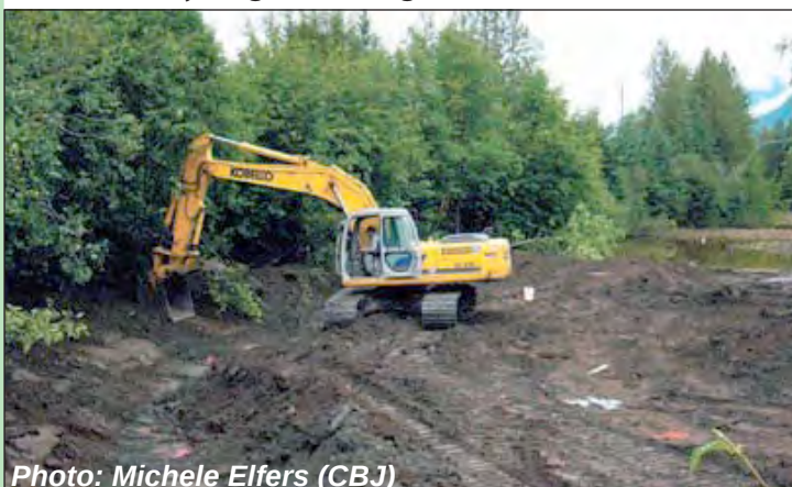
Digging outlet stream channel - July, 2006
