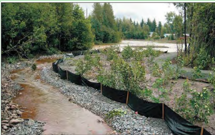
Alders transplanted along stream channel - 2006
