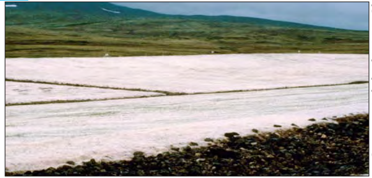
Excelsior matting on White Alice landfill - 1997
