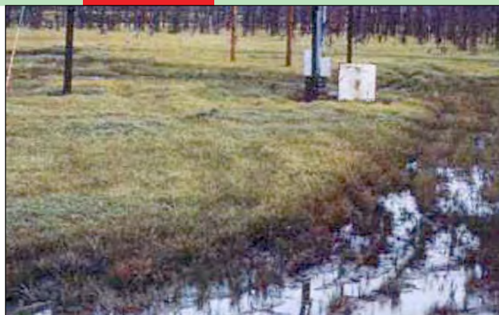
Girdwood switching station - September, 1995
