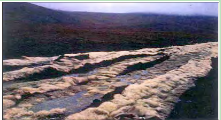
Trail after placement of excelsior mat - August, 1993
