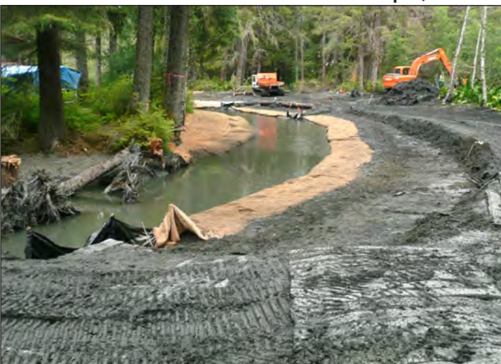
Late stage of channel rehabilitation - July, 2009
