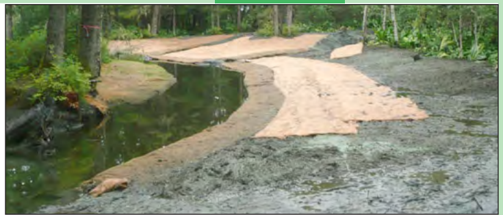
Floodplain seeded, coir fabric applied - July, 2009
