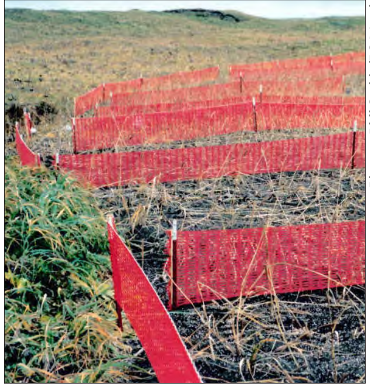
Newly sprigged roadway area protected from drifting sand using snow drift control fabric
