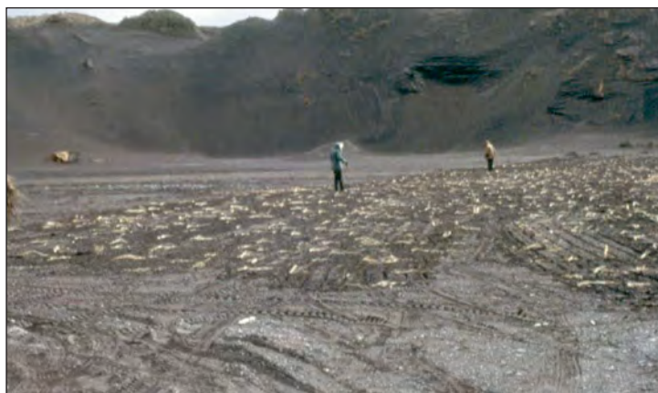
Sprigging the quarry area by hand - May, 1994
