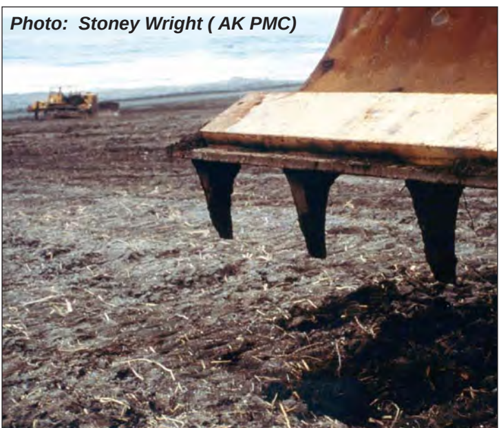
Mechanical trenching with 'Tiger Teeth' - May, 1987
