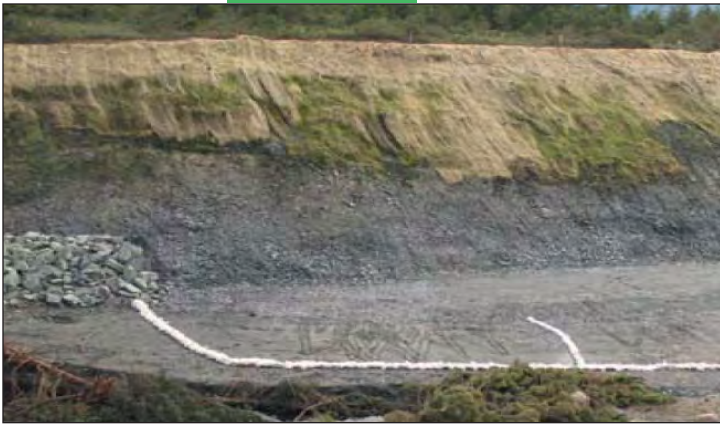
Cut slopes across from photo point 2 - August, 2008
