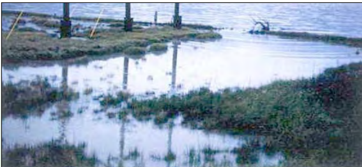
Access point 20-1A, at extreme tide - August, 1996
