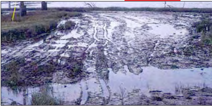
Access point 20-1A, prior to restoration - July, 1995
