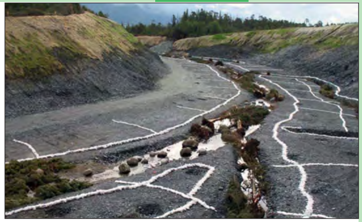
Constructed channel, looking upstream - July, 2007
