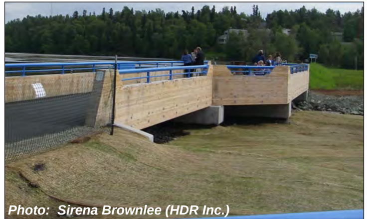
Erosion control matting near view platform - July, 2009
