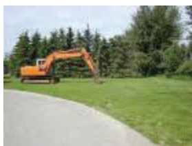
The work begins!
