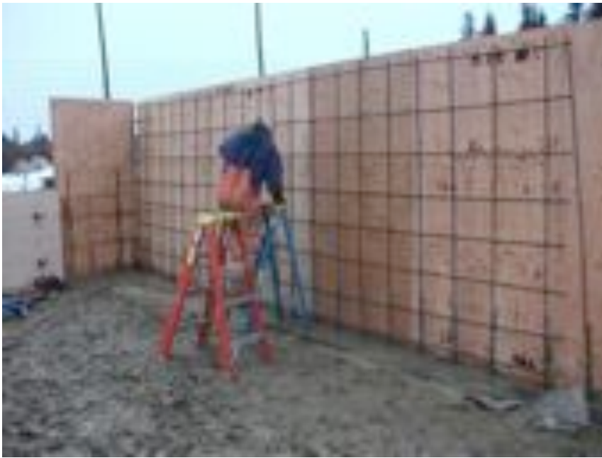
rebar grid, N wall
