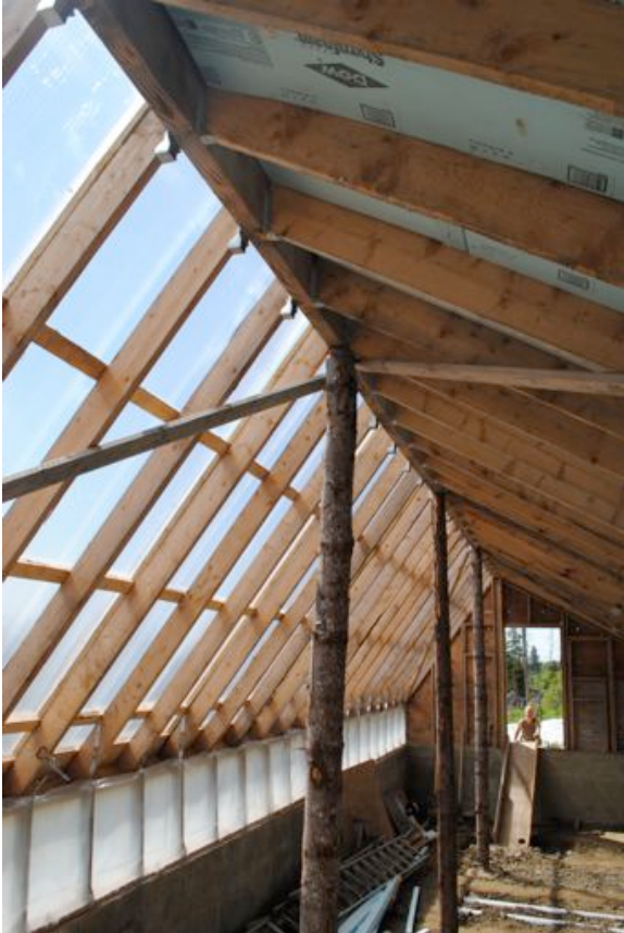
Interior construction spring 2012
