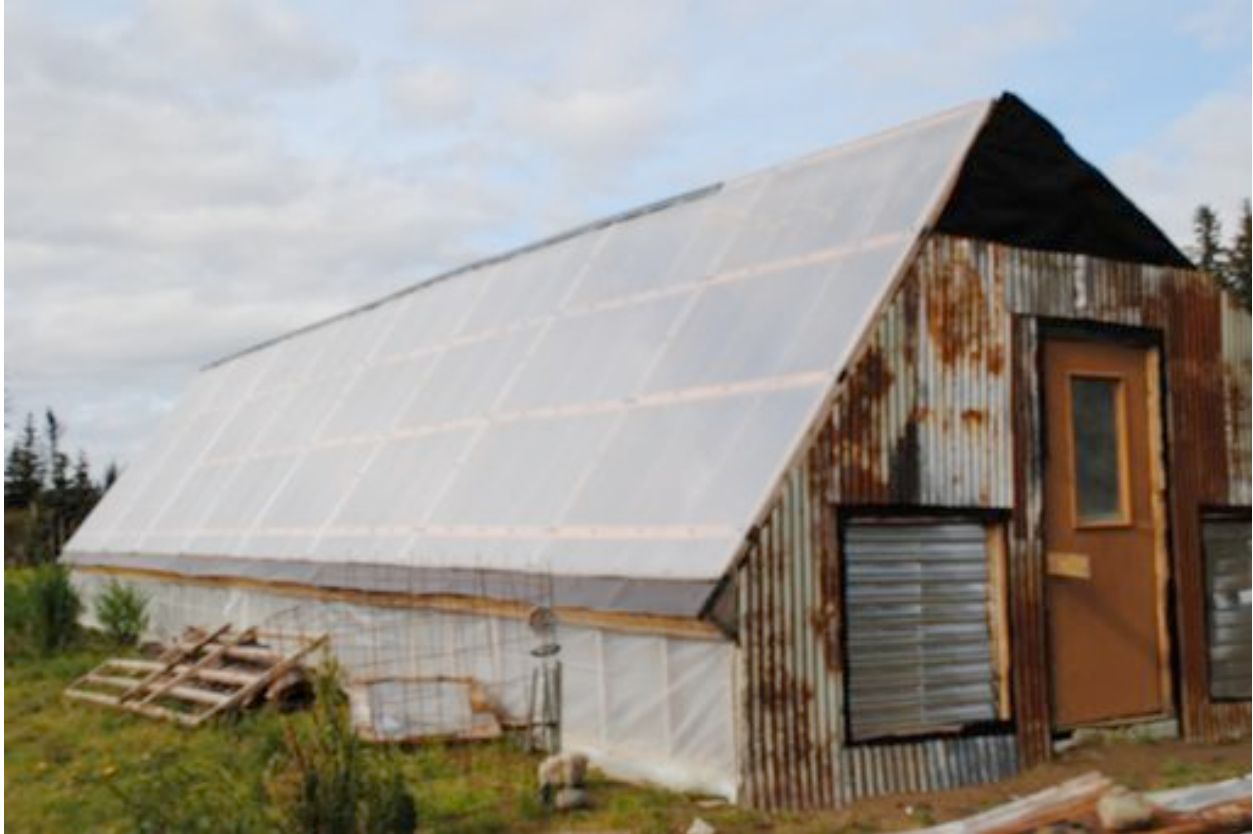
outside of greenhouse with recycled metal end wall siding
