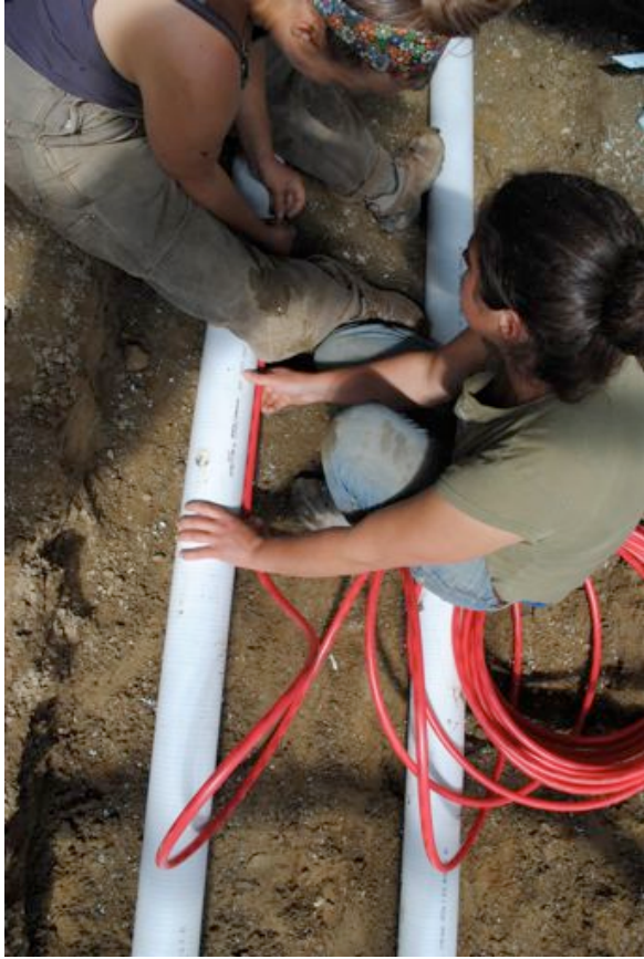
pex tubing for water transmission spring 2012
