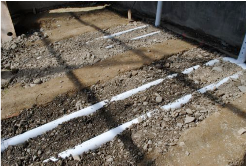
air pipes embedded in gravel below growing beds spring 2012
