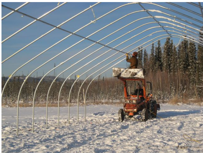
High tunnel construction November 2008
