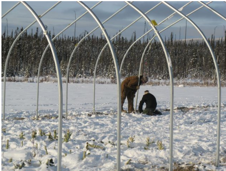
High tunnel construction November 2008
