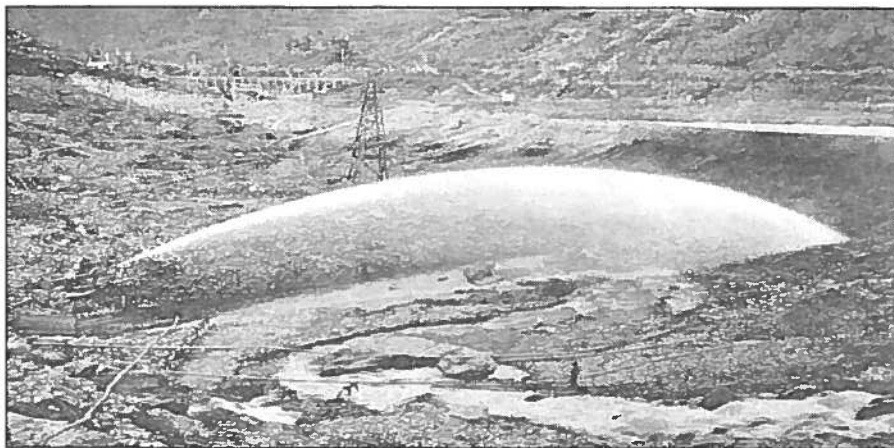
Figure 4. Example of Typical Hydraulic Operation in Alaska c.1905.
